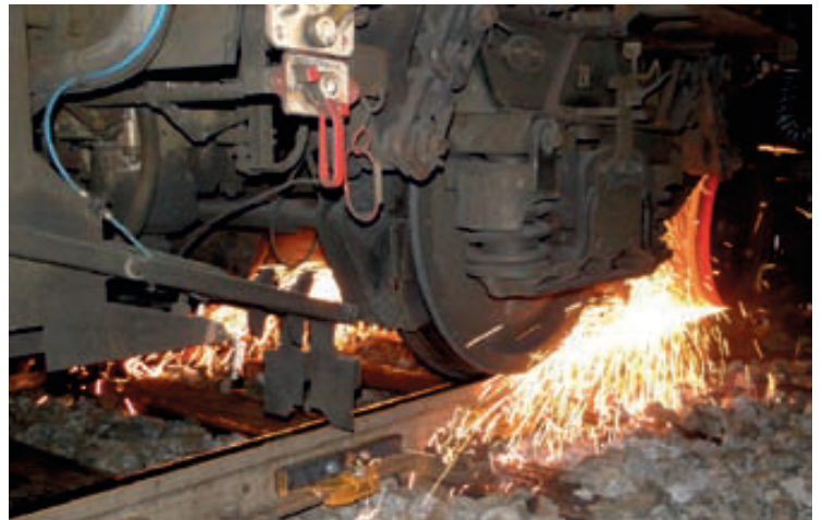
Rail grinding
