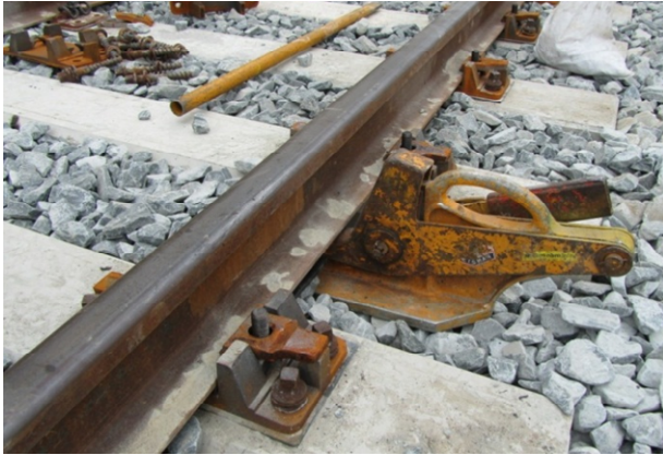
Figure 7 Jacking the rail
