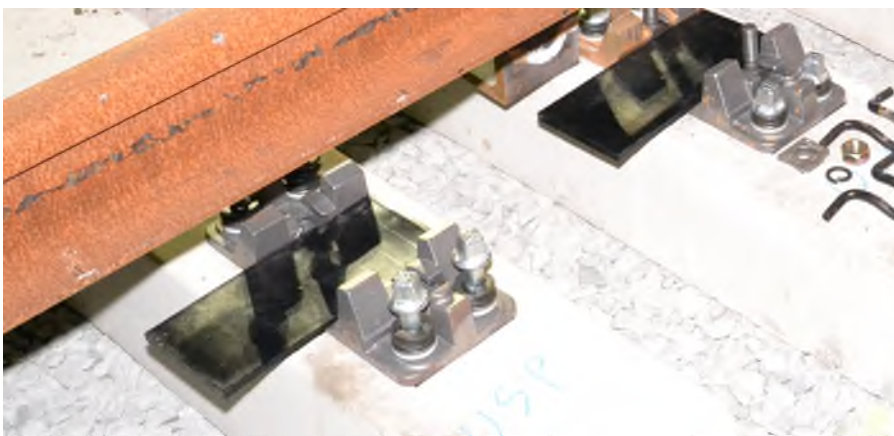
Figure 8 Fixing the ShimLift using existing bolts
