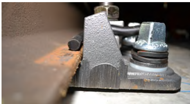
Figure 2 Front view of ShimLift type R rail fastening
