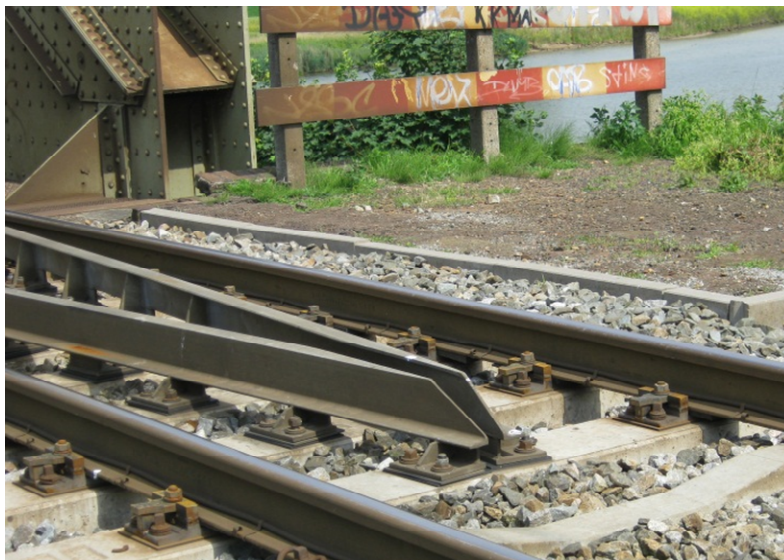
Figure 10 Shimmed derailment provision at transition with ShimLift
