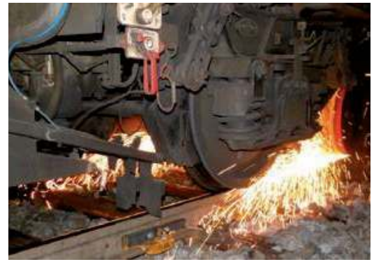
Rail grinding
